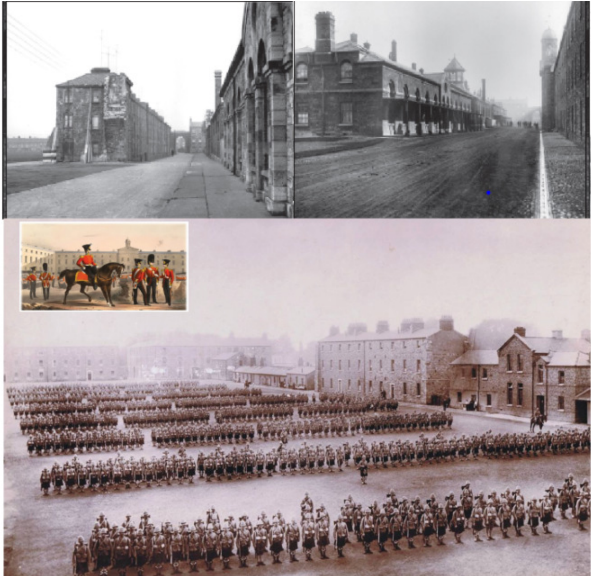
Figure 4.5: Images Showing Original Structures of Richmond Barracks
