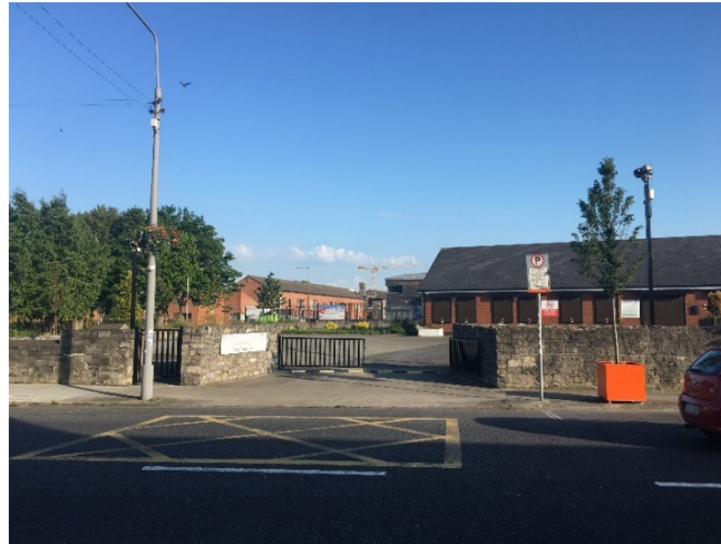
Figure 4.2: Entrance to Health Centre from Emmet Road
